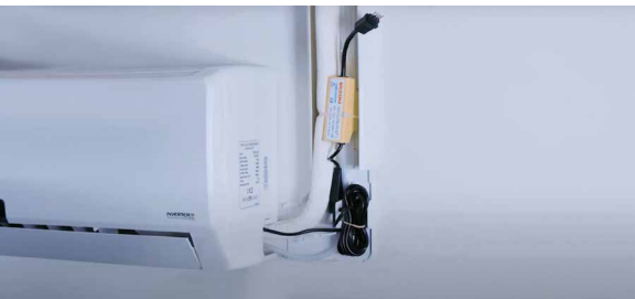
Solution with an externally incorporated condensate pump.
