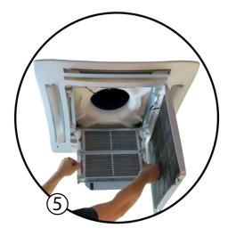
The aluminium filter can then be cleaned and washed in a domestic or industrial dishwasher or by immersion; The Crystall filter and the grille can then be repositioned and the SkySafe unit returns to 100% operation.
