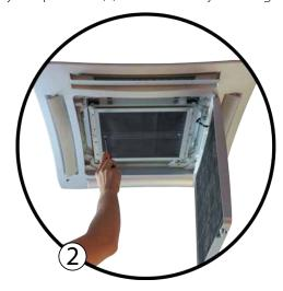
The Crystall filter is now easily accessible (3). Removing the fixing screw releases the filter holder frame which can be opened to pull the Crystall aluminium filters (4) out.
