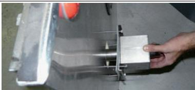
Place the upright in the 100 mm (3.9") opening made in the duct
