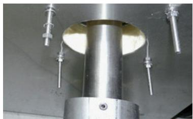
Tighten the support flange bolts to 7-8Nm (5-6ft), using the fastening elements supplied. If necessary, cut the bolts
