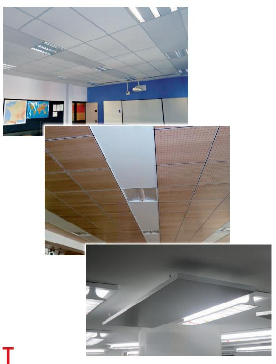
he panel can be supplied with hot or cold water: in the summer, it should be used together with a primary air system, as only sensible cooling is provided.
